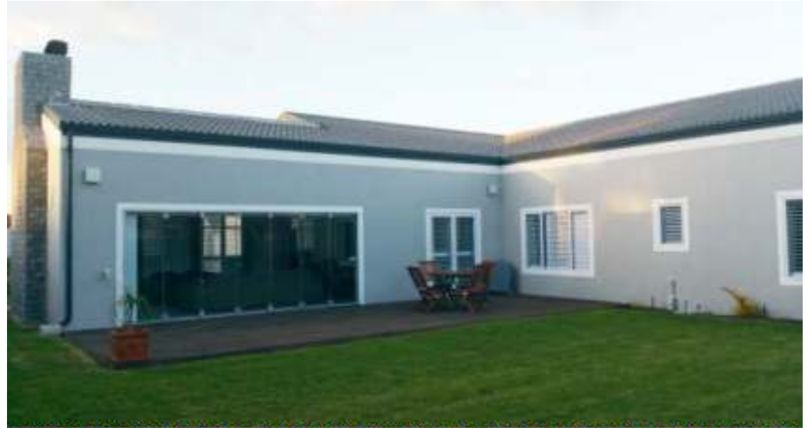
Solid Plastered Walls
