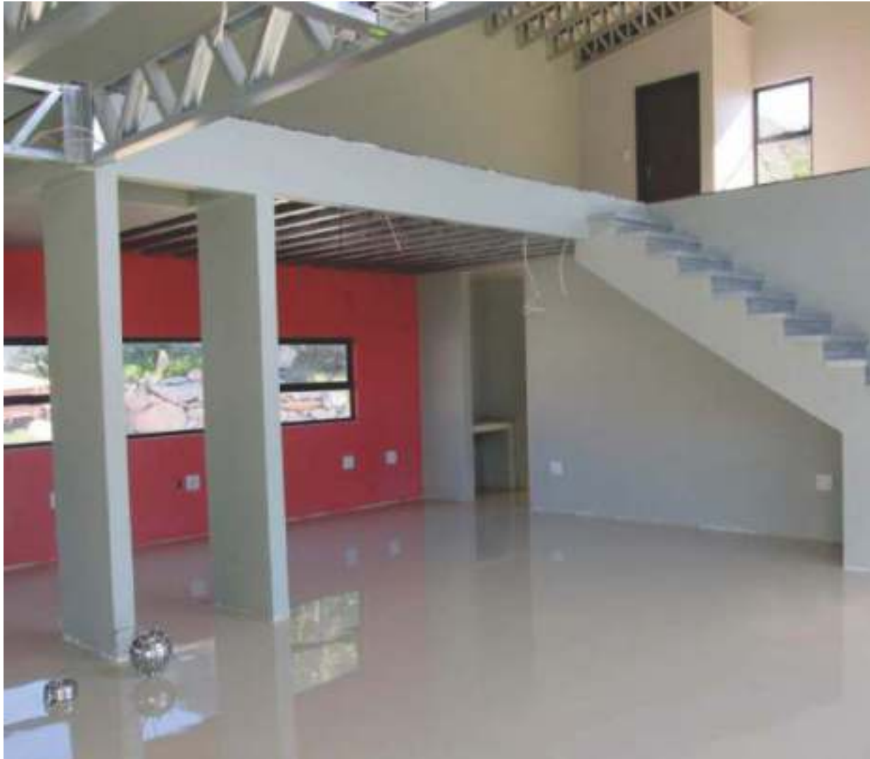
Completed Suspended Light Steel Frame Joist Floor
