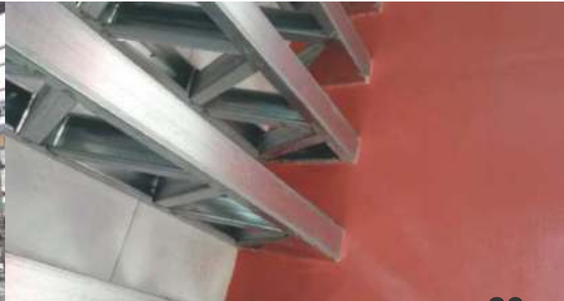
Finishing of Exposed Suspended Floor Joists
