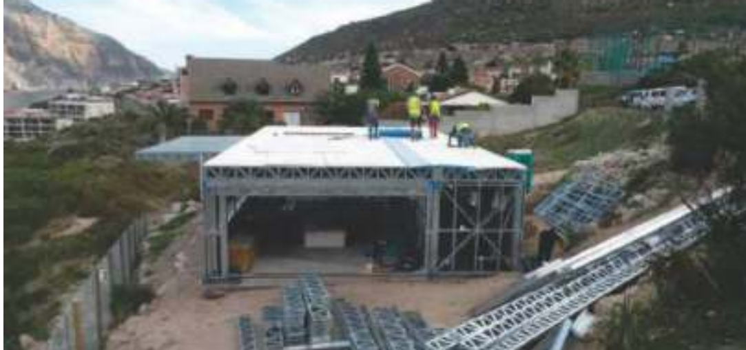
Installation of Floor Boards
