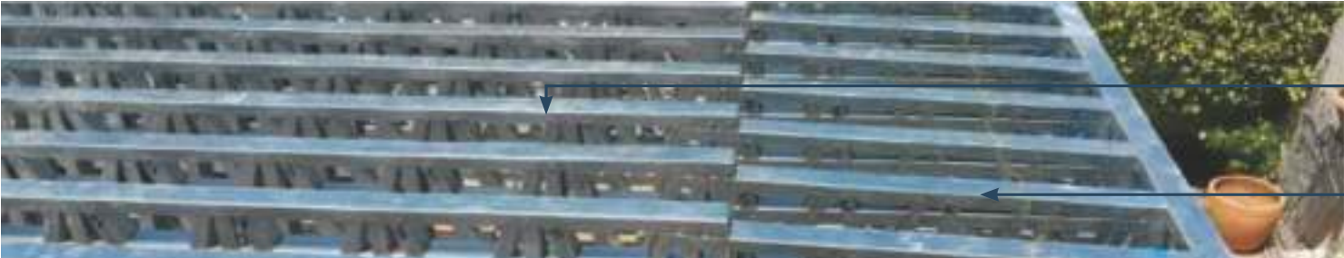
Light Steel Frame Cantilever Joist Floor
