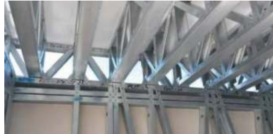
Light Steel Frame Joist Floor Anchored to Light Steel Frame Ring Beam
