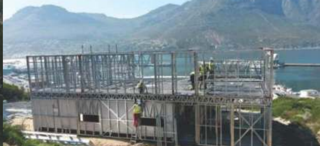
Installation of LSF Wall on LSF Joist Floor
