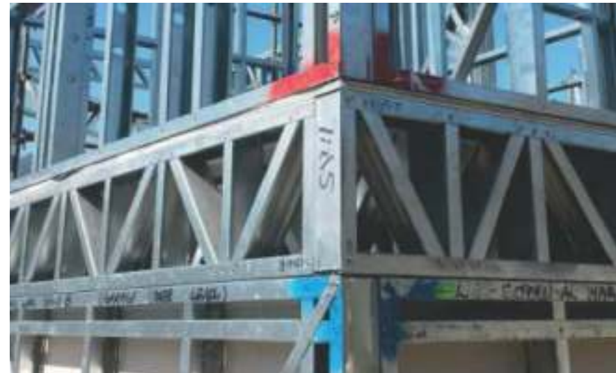
Light Steel Frame Ring Beam
