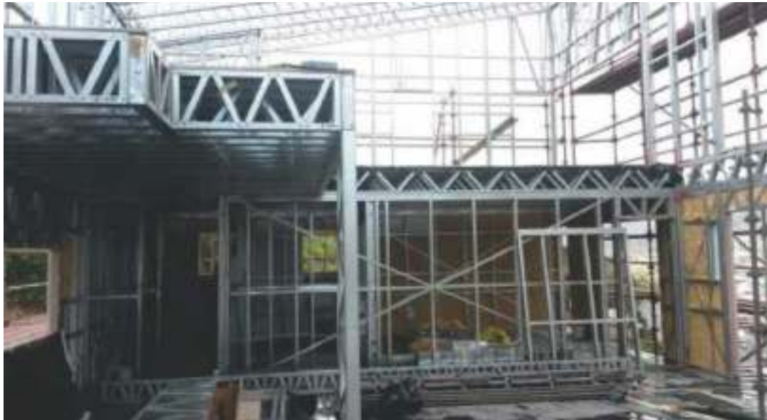
Suspended Joist Floor with Internal Cantilever
